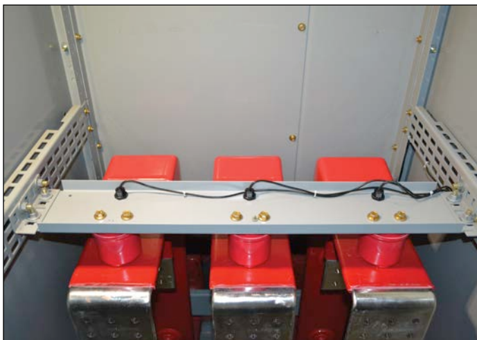
Figure 5.5-7. Typical Install for Continuous Thermal Monitoring Sensors
