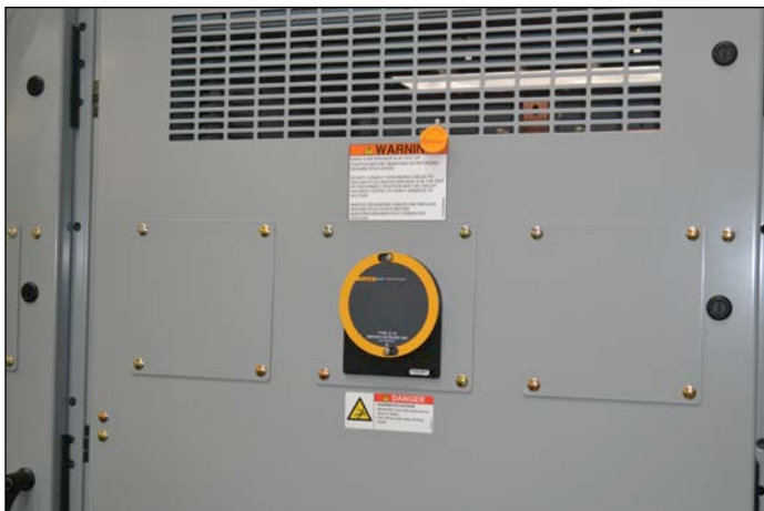
Figure 5.5-6. Typical Install for IR Window on Rear Door
