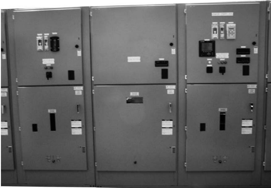
Front View—27 kV VCP-W Arc-Resistant Switchgear (Plenum Above the Switchgear is Not Shown)
