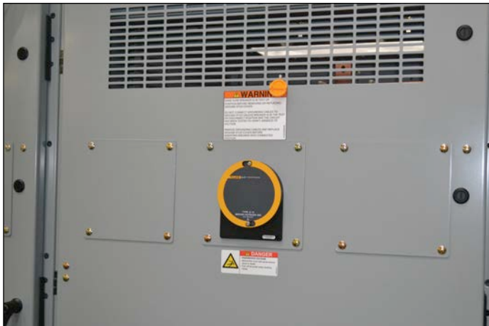
Figure 5.3-10. Typical Install for IR Window on Rear Door
