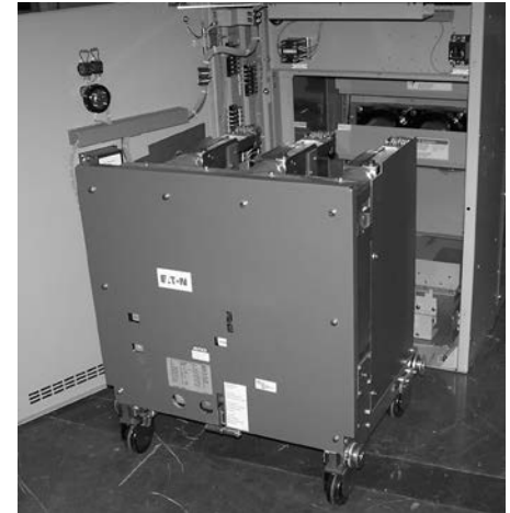
VCP-W Direct Roll-in Breaker with Fixed Wheels
