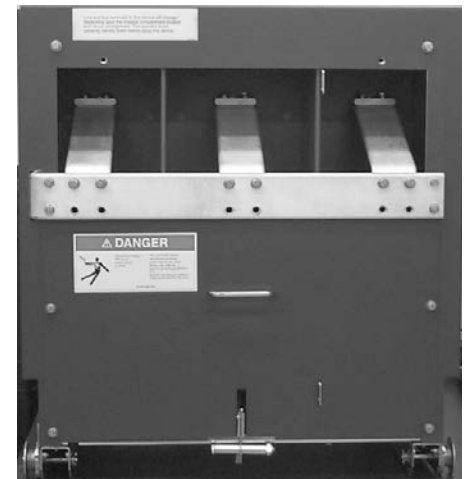
5/15 kV Manual G&T Device shown with Upper Terminals Grounded
