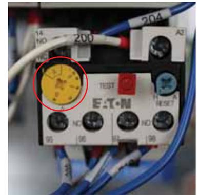
When an overload occurs, the 24 V control circuit power is removed via the NC overload relay contact (95-96) (see schematic). Both the VFD (M) and Bypass (B) contactors are disabled.
