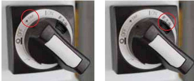
The VFD Logic and Keypad will have no power. The keypad will be dark.
